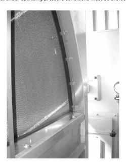
As a matter of course, rotor mounting will be aligned at the factory. Re-alignment may be necessary, however, depending upon the installation conditions. In this regard, please observe the manufacturer's operating instructions.
