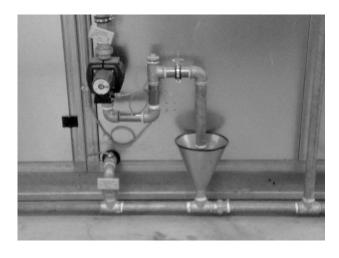
Horizontal drainage lines must have a sufficient diameter and slope gradient, as well as ventilation and bleed properties for fault-free water drainage.
