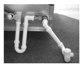
The siphon height should be accurately determined, dependent upon the pressure head.
