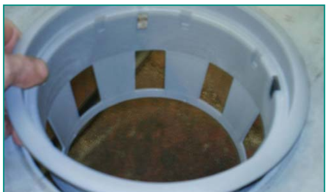
Figure 3: Place diffuser basket in opening
